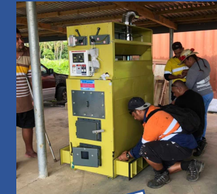
Assemble at the installation location
